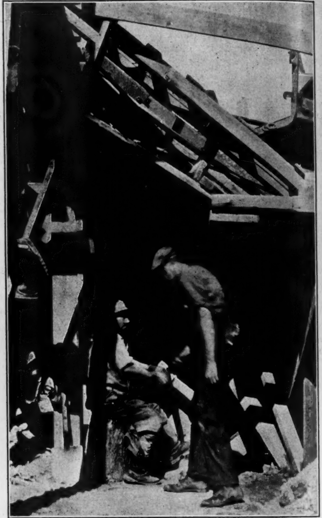
Manual Feeder Control of Material from Hopper to Elevator
